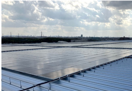
Installation of approx. 3MW solar panels
