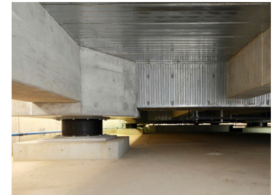
Seismic Isolators
