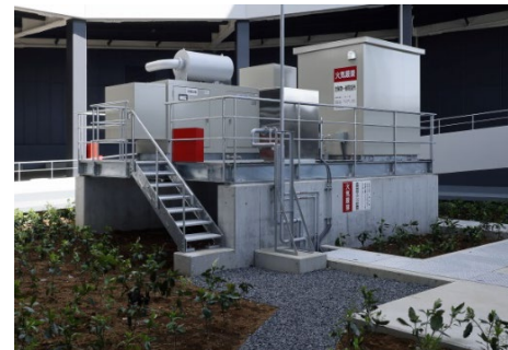
Emergency generators & large oil tank
