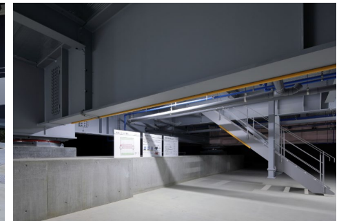
Advanced seismic isolator
